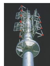
The rods on this broadcasting aerial are horizontal.
